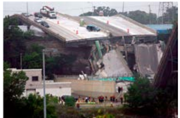
The 2007 Minnesota Bridge Collapse
